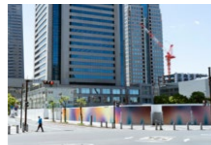
Construction wall design Photo: KATO Hajime
